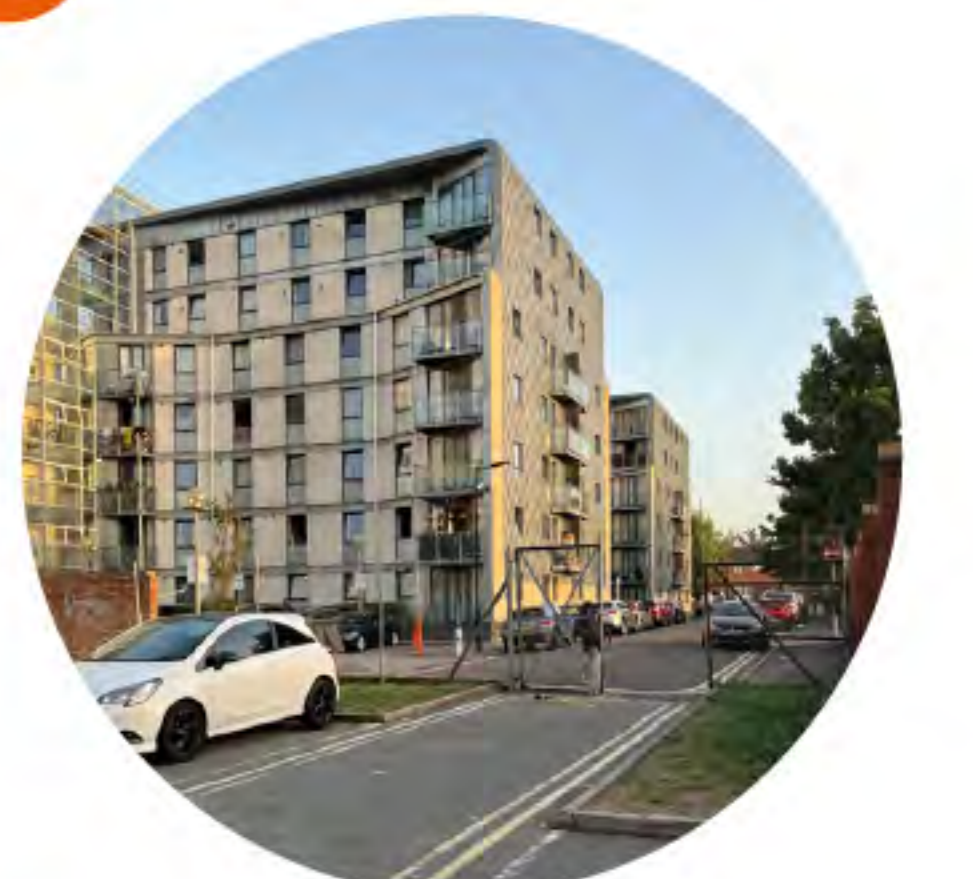
7 Old HSBC building
